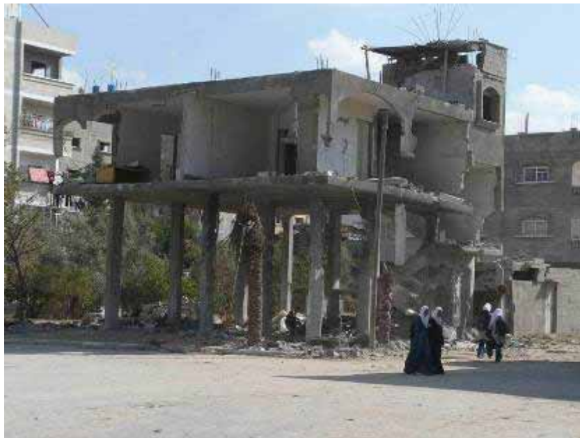
Salha family house, bombed on 9 January 2009 © AI
